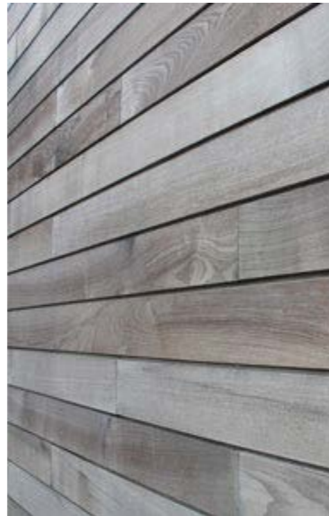
Weathered Brimstone ash cladding
